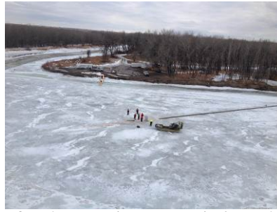
Containment and recovery on the frozen river: cutting slots in the ice to deflect the oil (Source: US EPA)
