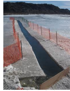
Containment and recovery on the frozen river: cutting slots in the ice to deflect the oil (Source: US EPA)
