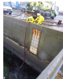
Fire brigade boom at the end of the wharf QR5 (left); pumping of trapped slicks by a vacuum truck (right) (Source: Cedre)
