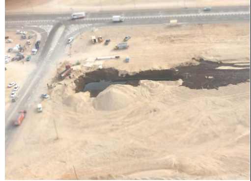
View of the breach in the Eilat-Ashkelon pipeline (Source: MCED)
