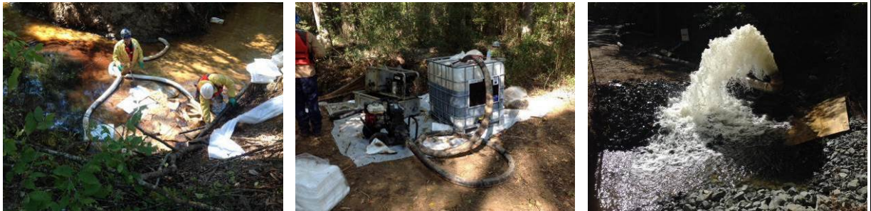
Manually collecting oiled sorbents (left); rope skimmer, pumping equipment and primary storage in IBC containers (+ ground protection using textiles) (centre); 29/10/14: pipe for flooding/rinsing upstream in the watercourse (right) (Source: US EPA)
