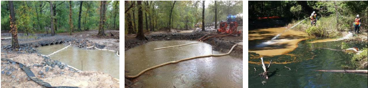
Containment by filter dams: bunds with pipes (left); Vacuum trucks for pumping floating accumulations between dams (centre); Concentrating the floating oil and directing it towards containment areas using hoses (right) (Source: US EPA)
