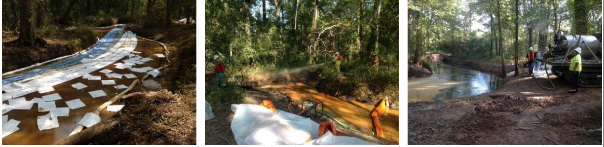
Collection using various types of sorbent (rolls, mats, pads) (left); localised rinsing of the banks using low pressure hoses (centre); pumping equipment deployed from small caterpillar track vehicles (right) (source: US EPA)
