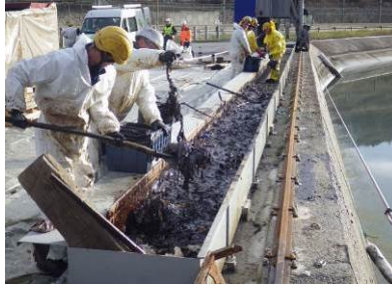
Low pressure rinsing of plastic liners with hot water (left); debris and fuel oil trapped in the screen of the Saint-Martin-de-la-Porte dam (right) (Source: Cedre)
