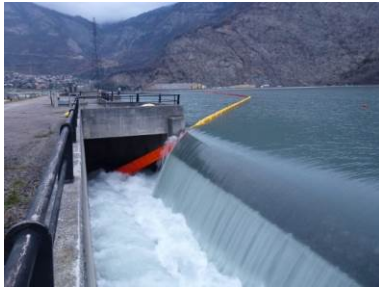
Testing the resistance of a boom to optimise the flow rate: the boom is drawn into the spillway at a flow rate of 80 m 3 /s (Source: Cedre)
