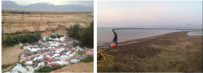
Laying mop sorbents in the Kinet Canal (left); boom set up on 9/12/14, in the port of Eilat (Gulf of Aqaba) (right) (source: MoEP)
