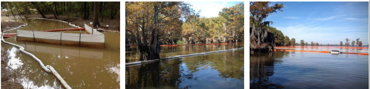
Containment/protection: in the creek, by floating booms, sorbent booms and oleophilic textiles on stakes (left); in the flooded area, by floating and sorbent booms (centre); at the mouth of Tete Bayou where it meets Caddo Lake, by rows of floating boom (with a drum skimmer between 2 sections of the 1st row) (right) (Source: US EPA)
