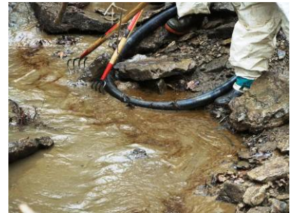
Remobilisation of infiltrated crude oil by scraping/tilling sediment (Source: wvxu.org)
