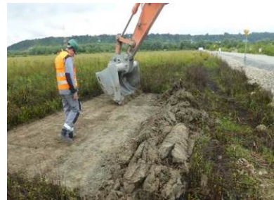
Skimming (oleophilic disc skimmer) accumulations of crude oil in a drainage channel (FOST responders) (left); Removing contaminated soil: ditch excavation (middle); Scraping the surface of grasslands (right) (Source: Cedre)
