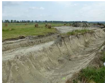
Skimming (oleophilic disc skimmer) accumulations of crude oil in a drainage channel (FOST responders) (left); Removing contaminated soil: ditch excavation (middle); Scraping the surface of grasslands (right) (Source: Cedre)
