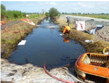
Skimming (oleophilic disc skimmer) accumulations of crude oil in a drainage channel (FOST responders) (left); Removing contaminated soil: ditch excavation (middle); Scraping the surface of grasslands (right) (Source: Cedre)
