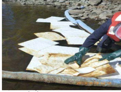
Final clean-up of banks: flooding with a deluge system (left); containment and recovery of released oil using sorbents (source: MDDELCC)
