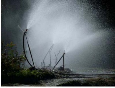
Final clean-up of banks: flooding with a deluge system (left); containment and recovery of released oil using sorbents (source: MDDELCC)
