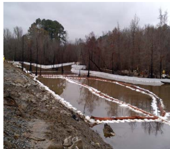
Sorbent mops on ropes, and viscous, sticky, weathered oil on the banks (left); containment booms lined with sorbent mops (middle); sorbent rolls taut between piles (right) (Source: US EPA)
