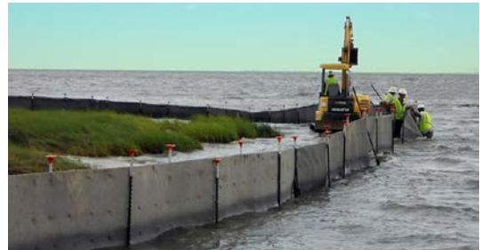
Ultra-Spill Fence ® being used to protect a sensitive shoreline - here at the edge of a marsh in Louisiana, during the Macondo spill, US 2010 (Source: http://www.spillcontainment.com )
