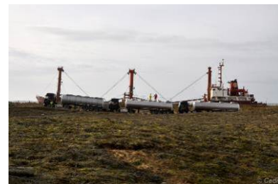
20th December 2011: defining access through the dune to set up the site for the bunker tank pumping operations by Smit Salvage and the evacuation of pumped fluids (Source: Cedre)
