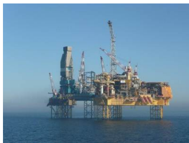
The Elgin rig, on the 27th March 2012 (2 days after the leak was reported) (Source: Total)
