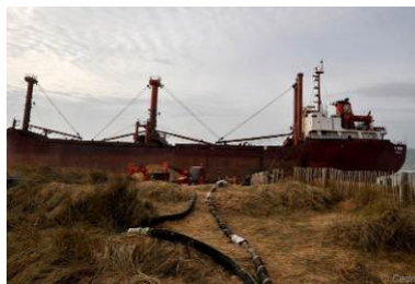
20th December 2011: defining access through the dune to set up the site for the bunker tank pumping operations by Smit Salvage and the evacuation of pumped fluids (Source: Cedre)
