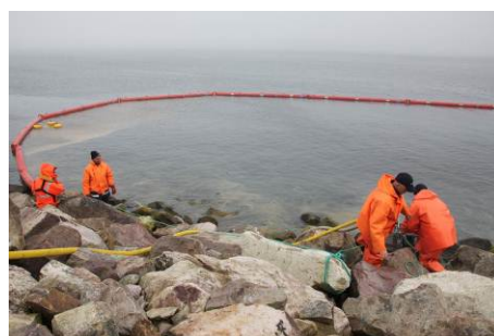
Containment and recovery at the foot of riprap (source: DTAM 975)
