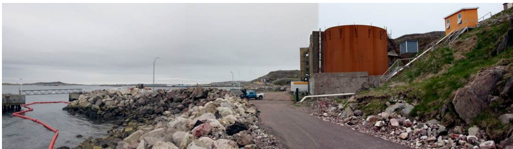
Site layout: right (orange) hut where the valves and pipes for filling tanker trucks are located. The heating oil ran down the slope, under the road, then through the riprap (source: DTAM 975)
