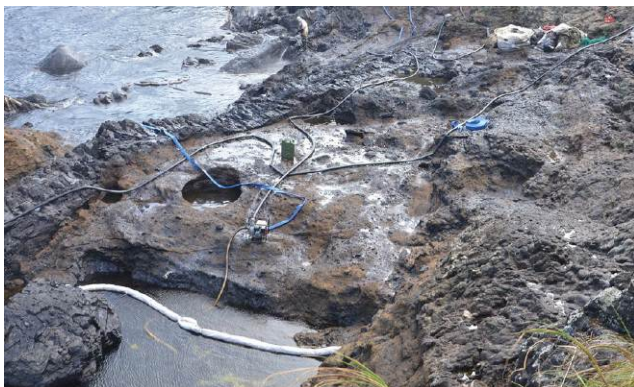
Clean-up site: rinsing and effluent containment operations (source: ITOPF)
