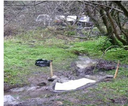
Laying sorbents at the incident site (source: Waikato Regional Council)
