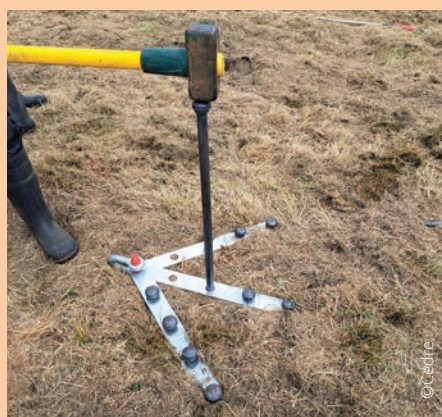
^ Ground anchor plate prior to trial
