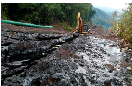
^ Digging drainage pits (left) and trenches (centre), using heavy machinery, as an emergency measure to reduce the spread of the oil from the breach in the pipeline; construction of earthen bunds at an outflow in the Coca River (right).
