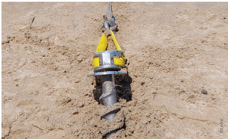
^ Screw anchor ripped out of the sand
