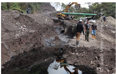
^ Digging drainage pits (left) and trenches (centre), using heavy machinery, as an emergency measure to reduce the spread of the oil from the breach in the pipeline; construction of earthen bunds at an outflow in the Coca River (right).
