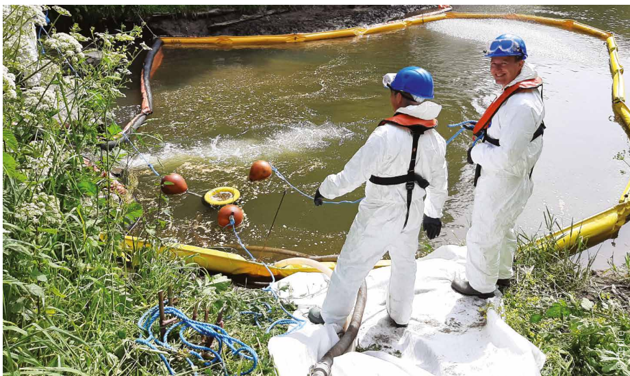
▲ Deploying a protective boom as part of a practical exercise in inland waters
