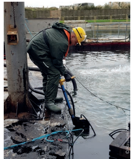
▲ CCME participant handling a handheld brush skimmer during the training course.
