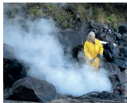
High pressure-hot water cleaning on rip-rap shoreline
