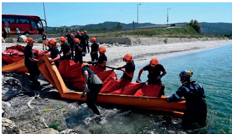
^ Coordinated installation of a boom on the Étang de Berre
