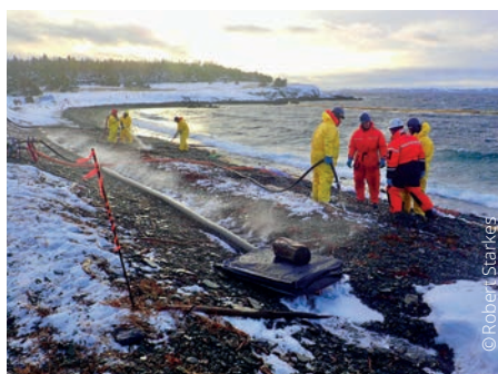
Low pressure flushing on oiled shoreline during a winter response
