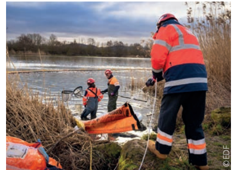
^ Containment of the oil residues and assessment at the boom installed at the site's discharge station
