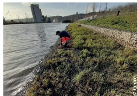
▲ View of the upper part of the north bank
