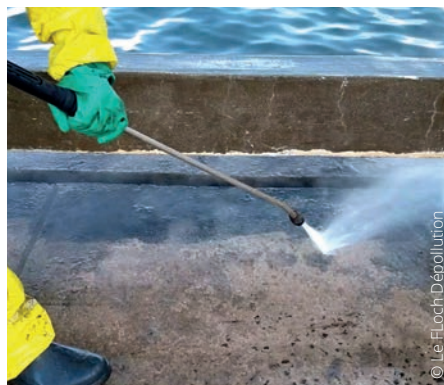
^ High-pressure cleaning of a dock
