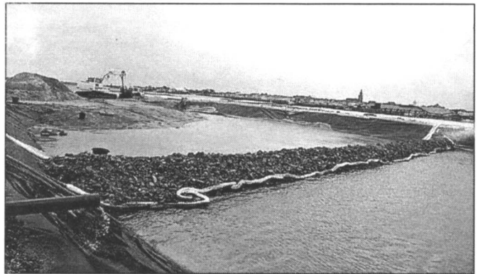
Figure 12. The pools separated by the stone wall/mound. The temporary storage facility for dredged sand.
