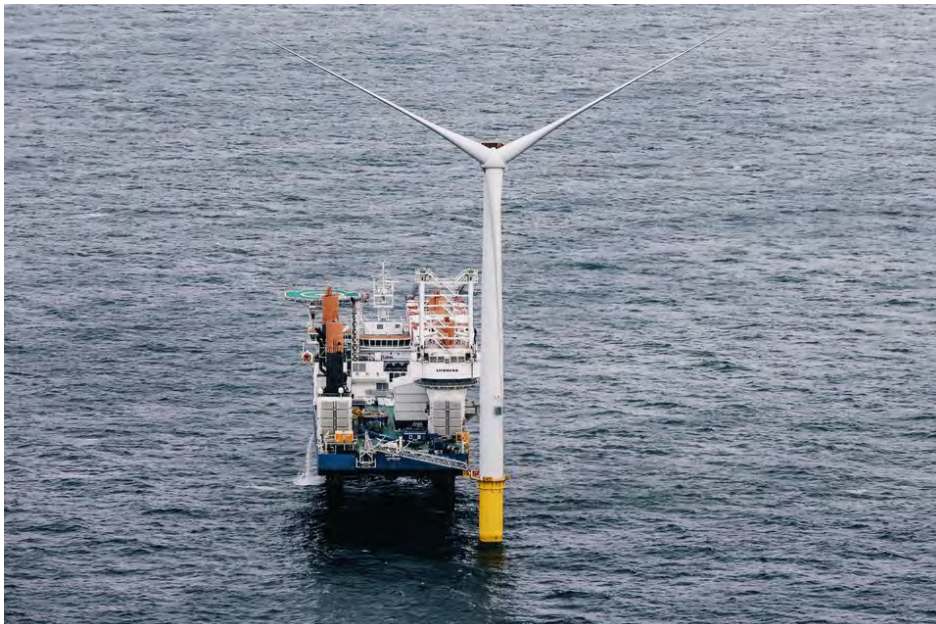
Figure 9 – Maintenance of a wind turbine at sea. De Standaard, 5 Oct 2023 © Kenzo Tribouillard.
