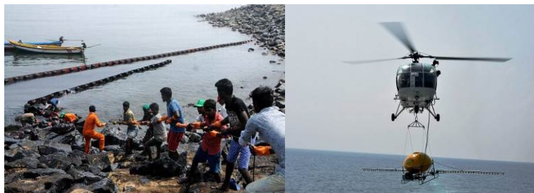
09/02/2017: Responders (ICG and volunteers) mooring booms to prevent the oil from spreading (Source: B. J. Ramalingam, RR) (left); 03/02/17: Applying chemical dispersants by helicopter (Vikoma TC3 dispersant system) (Source: PTI) (right)
