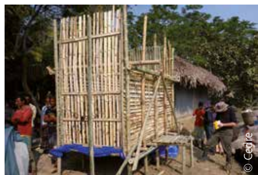
Draining oiled vegetation in a bamboo storage cage with an oil-tight base liner
