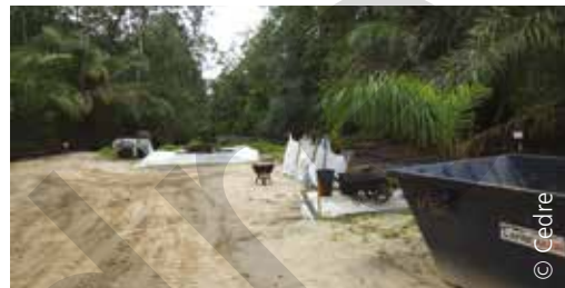
Temporary waste storage and sorting site
