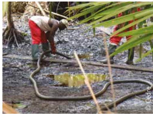
Removing pockets of oil by suction using a vacuum truck
