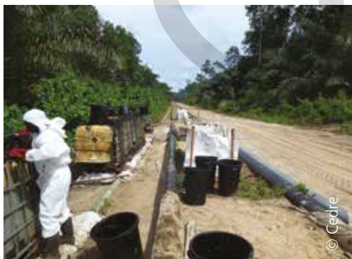
Traffic lane alongside a pipeline, clean-up site access and primary storage
