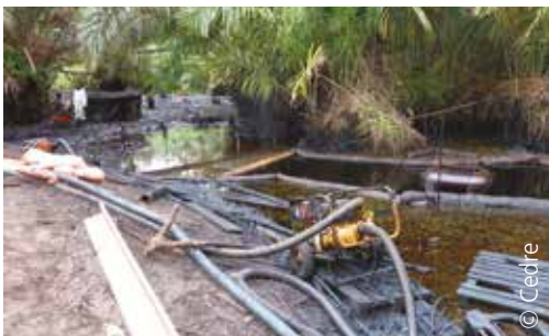
Recovering the oil using a disc skimmer
