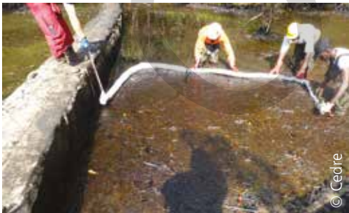
Containing the pollutant using a bottle boom
