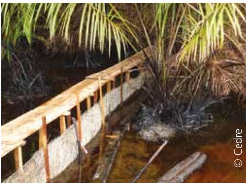
Filtration system filled with palm tree fibres installed under a walkway
