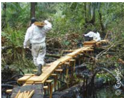
Extending an existing walkway
