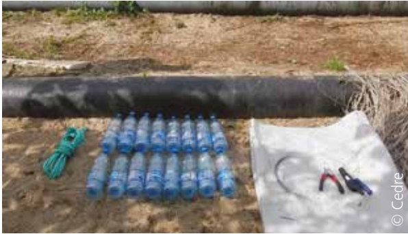
Preparing the necessary materials, laying the strip of geotextile on the ground, laying the rope then the bottles
