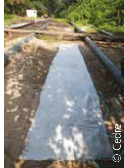
Preparing the necessary materials, laying the strip of geotextile on the ground, laying the rope then the bottles
