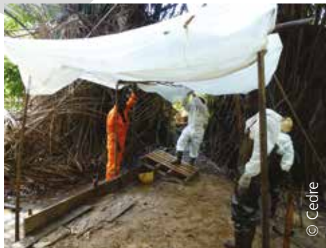
Provisional shelter at a clean-up site
