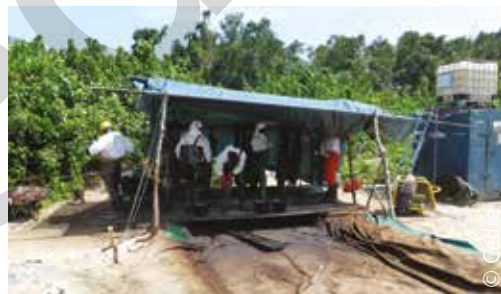
Decontamination area equipped with a pressure washer connected to a water supply (placed at a height on a container)
