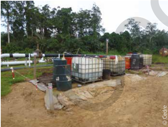
Fuel storage area
