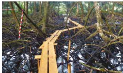
Walkway above aerial roots
