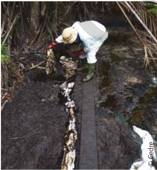
"Suit mops" laid at a drainage network
