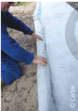
Rolling the geotextile around the bottles
