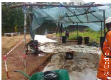
Full view of a decontamination area
