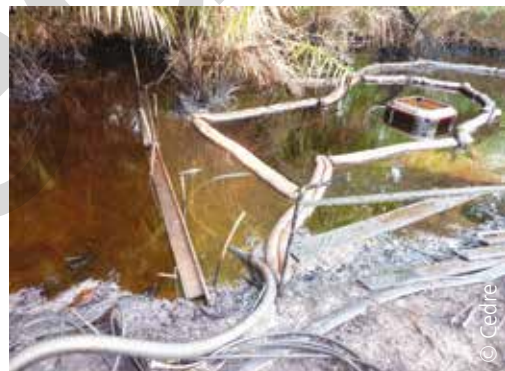
Containment using an alveolar structure
