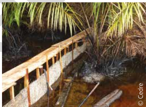
Attaching the wire casing under the walkway
