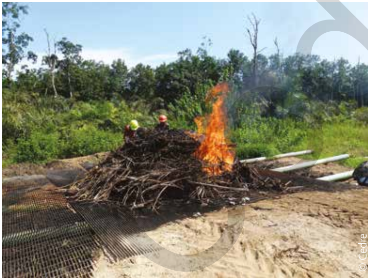
Lighting the fire and incinerating oiled vegetation
