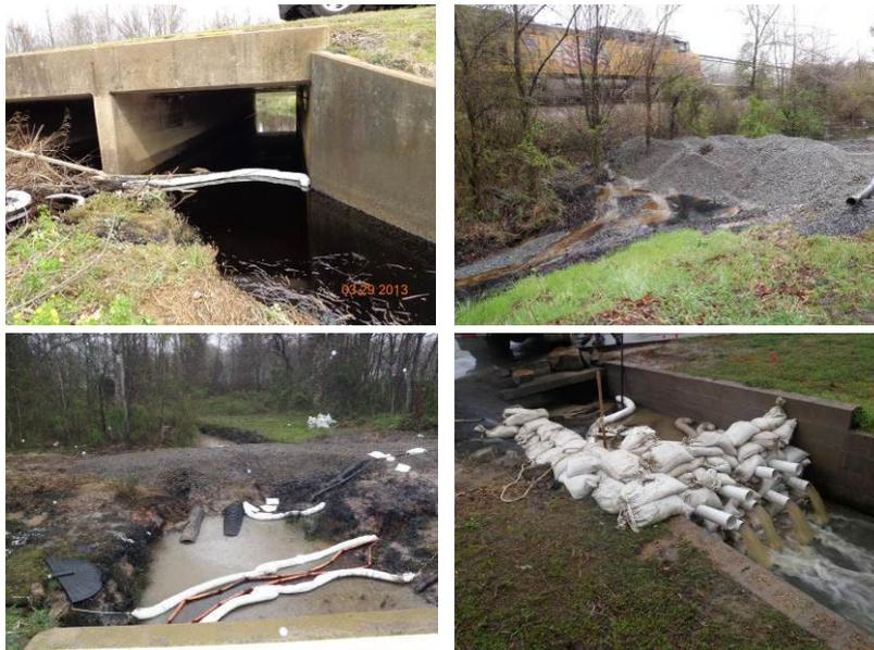
Various forms of containment of Wabasca heavy crude on the water: by sorbent booms (top left); by backfill (top right; note the penetration of the oil through the gravel); by filter barriers (bunds with pipes) in rivers (bottom left) and in a storm drain (bottom right) (source: US EPA).
