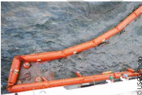
Using a boom to concentrate the oil and promote its recovery, Gulf of Mexico spill (2010)
