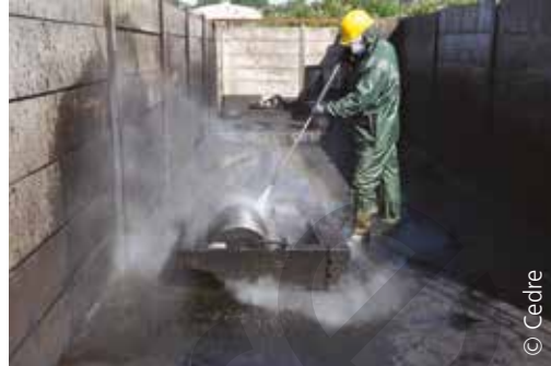
Cleaning a skimmer at a suitable site
