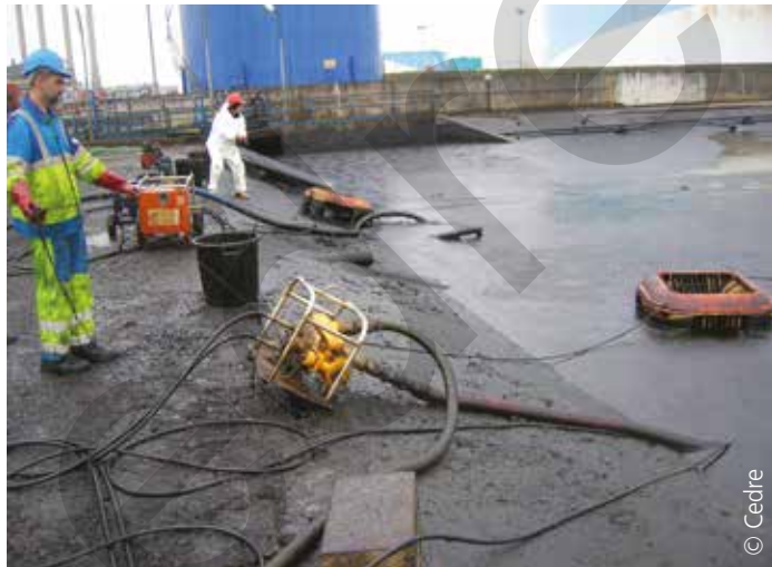
Skimmers with separate pumps
