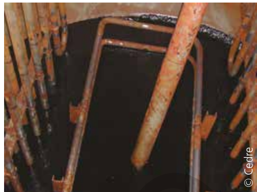
An onboard tank fitted with heating coils
