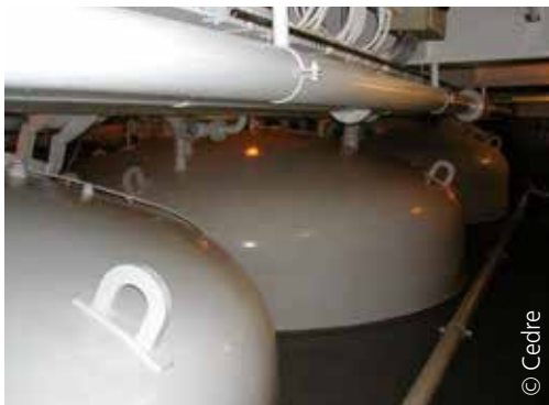
Storage tanks onboard a recovery vessel
