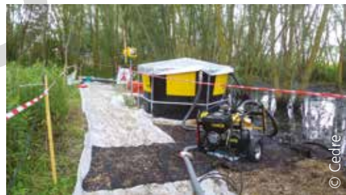
Separate transfer pump beside a storage and settling tank
