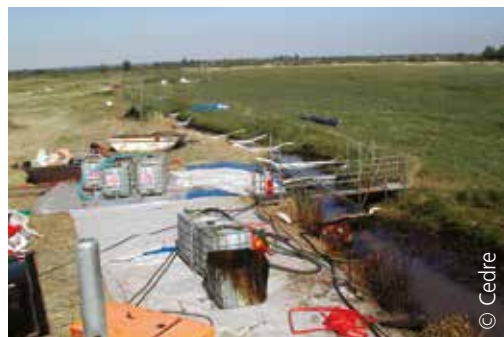
Containment and recovery in a watercourse and storage of the recovered oil
