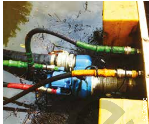
Fittings on hydraulic and transfer hoses
