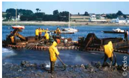
Recovering washing effluents on the shoreline
