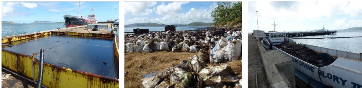
Left: storage of the fuel oil recovered on board and around PB103, before being transferred to the tanker Obama (in the background); Centre: bags of oiled waste; Right: barge mobilised to evacuate solid waste (source: Cedre)
