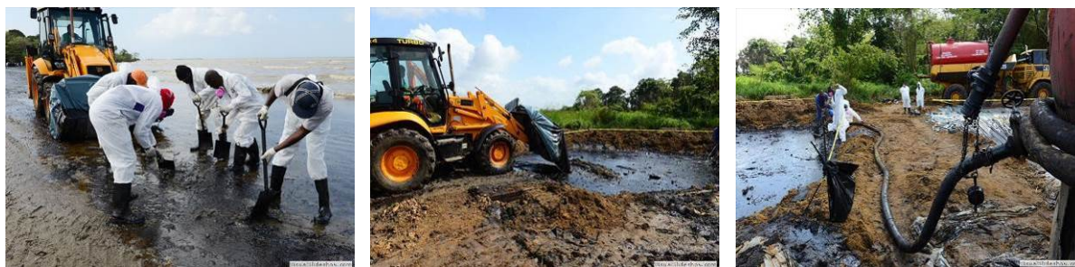
Organisation of the shoreline recovery chain: Left: manual collection with support from mechanical equipment; Centre: primary storage (lined pit) temporarily established on the back beach; Right: pumping of fuel oil (vacuum trucks) prior to transfer to the treatment site (source: www.petrotrin.com/ )
