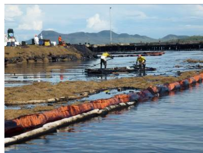
Mid-December: manual recovery using natural sorbents (rice straw) (source: Cedre)
