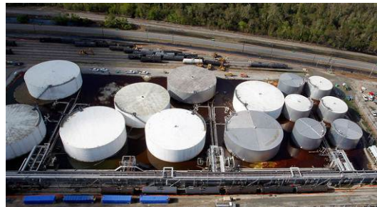
13/09/2012. Leaking tanks, at the Stolthaven New Orleans LLC chemical plant (Braithwaite), following Hurricane Isaac (Source: D Grunfeld / Times-Picayune DR)
