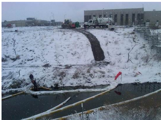
Containment, at the edge of the bank, of gasoline seepage with an earthen dam and booms (Source: US EPA)
