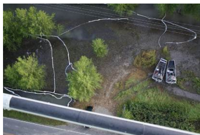
Containment using sorbent booms along flooded banks (left) and in trenches along the south bank (right) (Source: USFWS)
