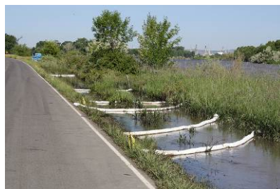
Containment using sorbent booms along flooded banks (left) and in trenches along the south bank (right) (Source: USFWS)
