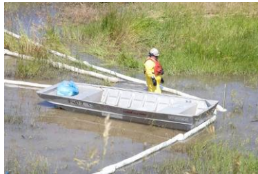
Maintaining sorbent booms using a jonboat (Source: USFWS)
