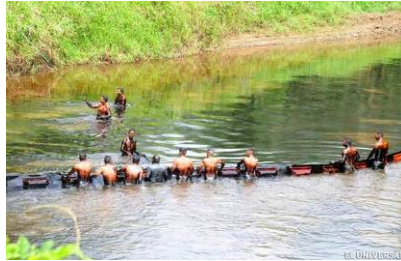
Volunteers deploying a permanent boom (source: El Universal)
