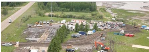
Aerial view of Cottonwood onsite command centre, set up by Plains Midstream -June 2012 (source: Plains Midstream)
