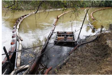
Containment (floating and sorbent booms) and recovery (oleophilic drum skimmer) (source: Agencia Venezolana de Noticias)
