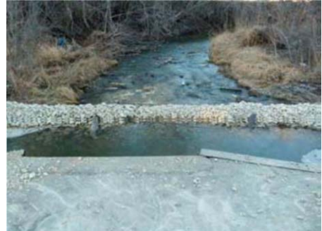
A limestone filter dam across Lime Creek downstream of the spill point. (source: KDHE)
