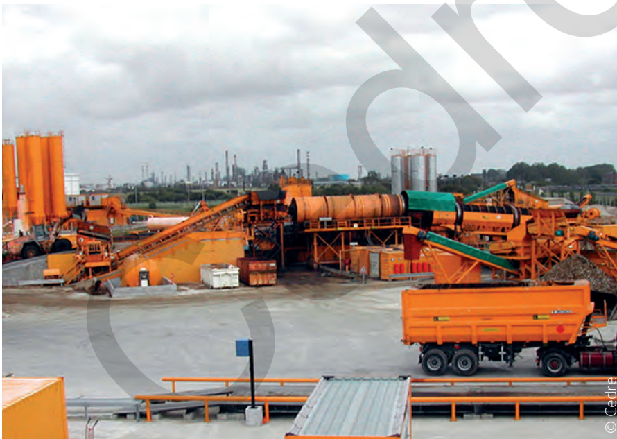
Waste treatment centre built during the Erika disaster: sediment washing station (Brézillon).
