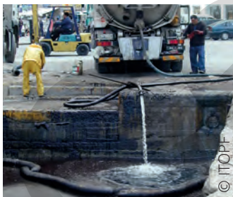
Release of water into a containment area after settling in a vacuum truck
