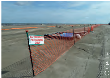
Worksite organised into zones with an access corridor before entering the "operations" zone and a decontamination area
