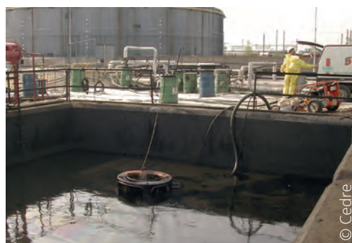
Pre-treatment operations carried out on the industrial site: settling/separation of oil and water collected in the estuary for oil recycling
