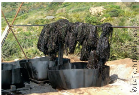
Example: sorbent mops (or "pom poms") drying on site for reuse
