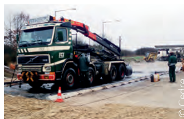
Decontaminating a vehicle before it leaves the storage site
