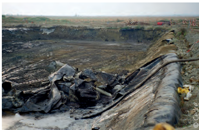
Dismantling of a long-term storage site, removal of tarpaulins lining the base and sides of a pit
