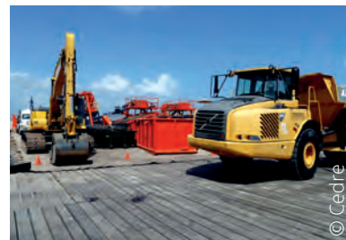
Mi-SWACO sand cleaning station, installed on a wooden platform on Grand Isle beach, Louisiana
