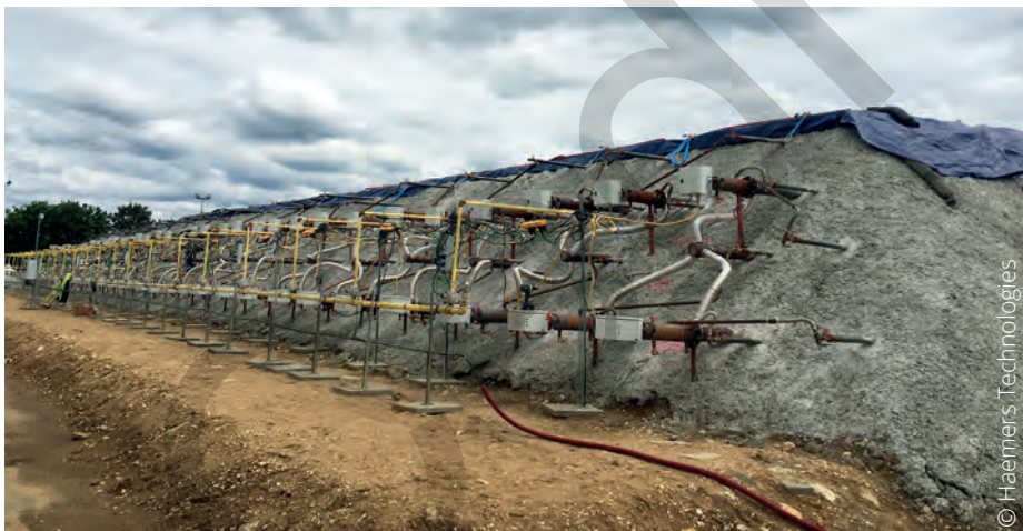
Treatment of polluted soil by thermal desorption - Pile in the process of being treated
