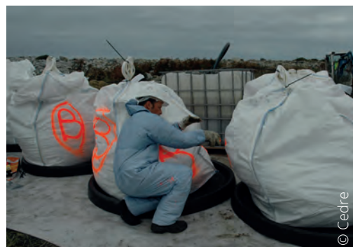
Primary storage in big bags on top of a custom-made retention system
