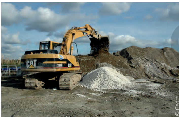
Lime treatment by mechanical mixing
