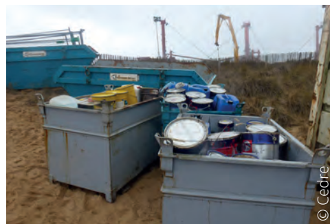
Primary storage site for chemicals from the dismantling of a grounded ship
