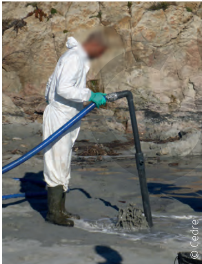
Remobilising pollutant trapped in the sediment using a low pressure water jet (flushing technique)
