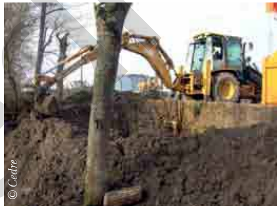
Complete blockage by cofferdam at the outlet of a road drain in which oil had accumulated
