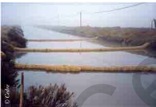
Protecting a stream in Bourgneuf Bay using straw-filled mussel nets
