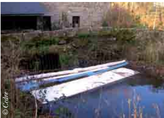
Sorbent boom and mat at entrance to mill spillway
