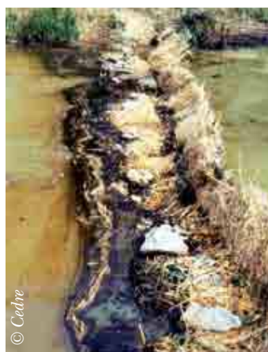
Barrier made of mesh and straw, Loire 1999
