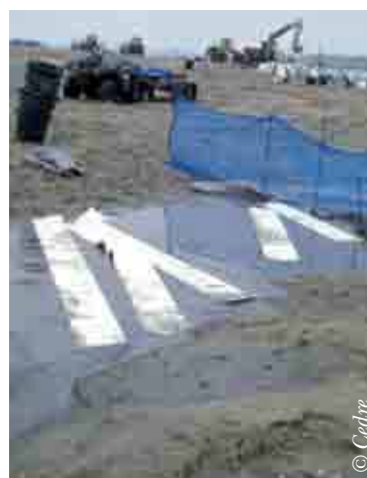
Recovering washing effluent using nets and sorbent pads
