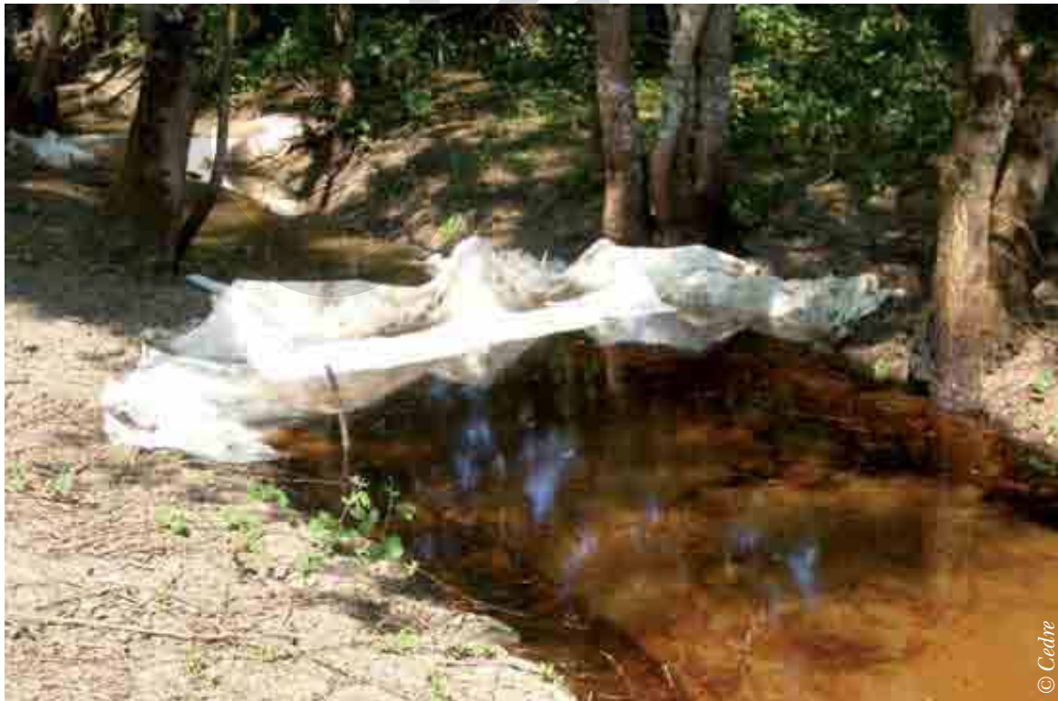
Filter barrier made of straw, sorbent and geotextile installed on a stream polluted with crude oil, Ambès 2007
