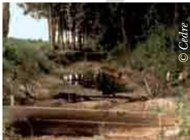
Blocking off an oiled trench liable to flooding
