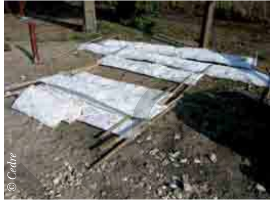
Channel filter barrier built in advance, Ambès 2007
