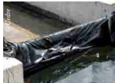
Run-off blocked in a concrete outfall using planks and plastic sheeting
