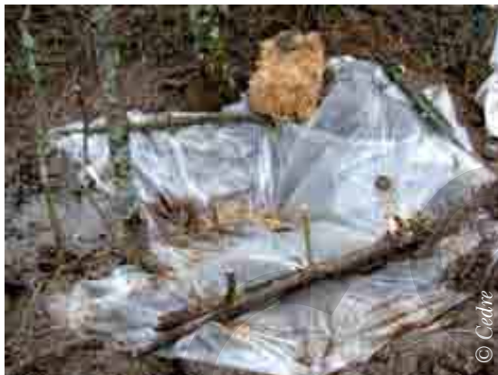
Complete blockage of a trench by a bund and plastic sheeting
