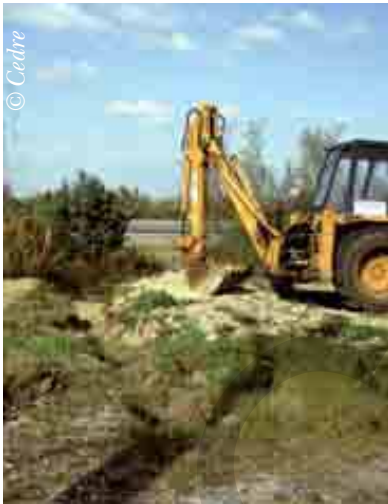
Blocking off a trench after a road tanker had overturned
