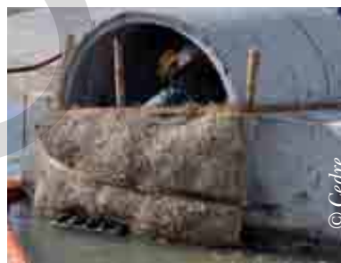
Mesh and straw device attached by ratchet straps and posts
