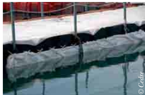
Permanent containment around a pontoon using geotextile attached to bamboo trellis
