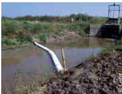
Protecting a stream using a filter barrier and sorbent fibres
