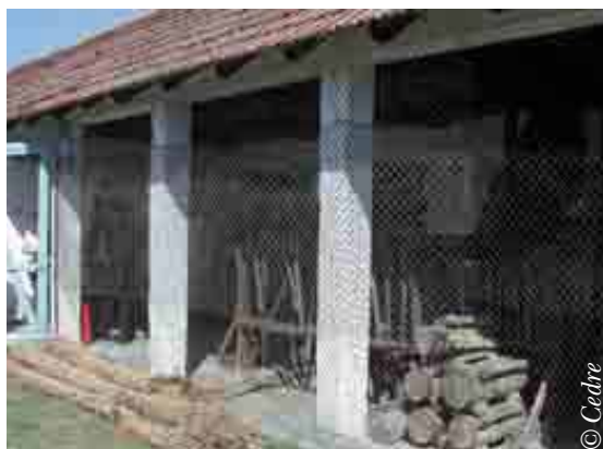
Stockpile of materials to build barriers, Romania 2007
