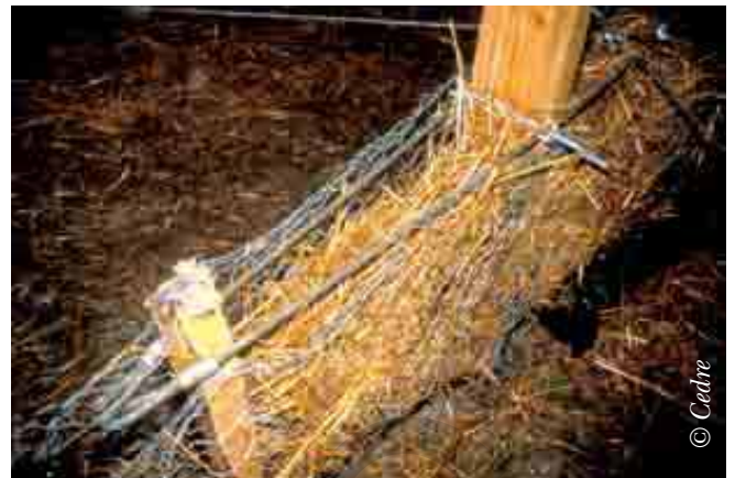
Protecting the sea inlet at Le Croisic, which feeds into Guérande salt marshes, using a straw filter barrier
