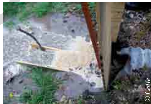
Underflow barrier made of plywood placed on wooden blocks in a stream
