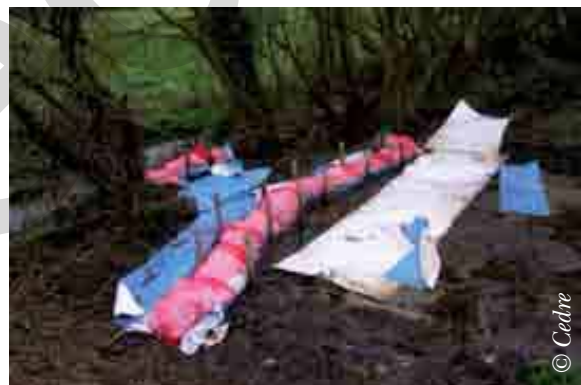
Reinforced measures: sorbent pads and loose sorbents in a plastic mesh pod held in place with wooden stakes
