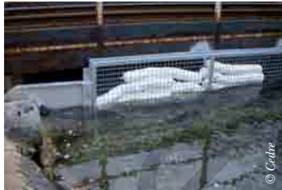
Retaining a spill at a discharge outlet using a filter cartridge
