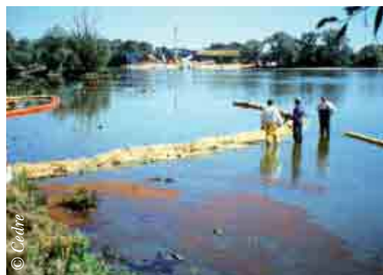
Straw filter barrier required to overcome the limitations of the boom already deployed
