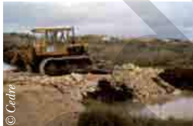
Closure of a stream at risk using sediment
