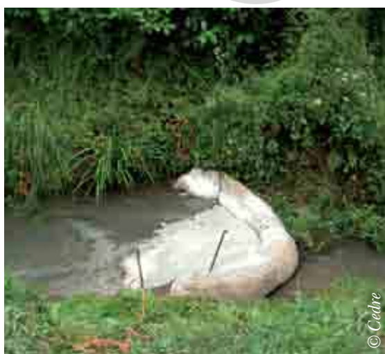
Barrier made of net, straw and sorbent fibres, 2011
