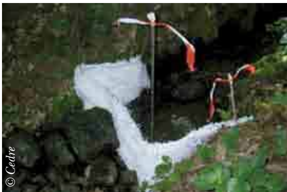
Filter cartridges made of mesh and filled with loose sorbents laid just downstream of the wetland clean-up site (←) and in a stream (→), with a sorbent pad
