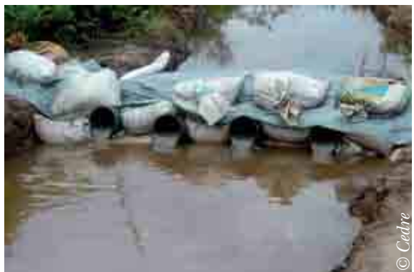
Barrier with angled pipes laid in an outfall (←) and in a stream (→)
