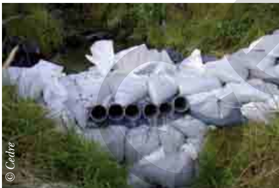
Barrier made of bags of sand and PVC pipes
