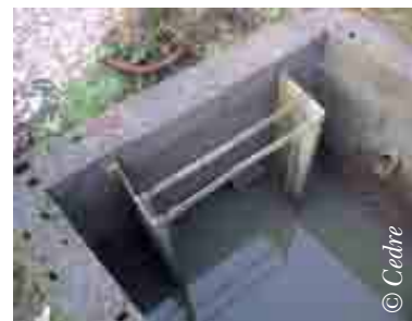
Track into which a perforated metal filter and sorbent fibres can be inserted
