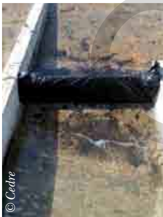
Underflow barrier made of planks and plastic sheeting in an outfall
