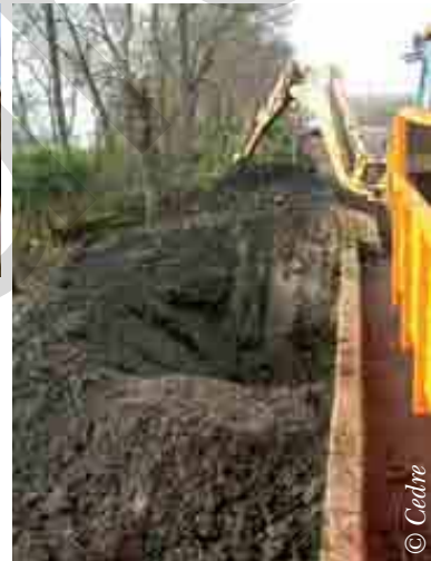
Building an earthen dam at a polluted drain outlet
