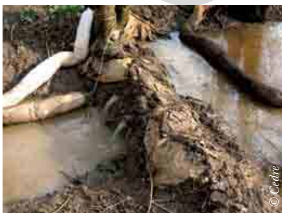
Earthen dam with angled pipes and sorbents
