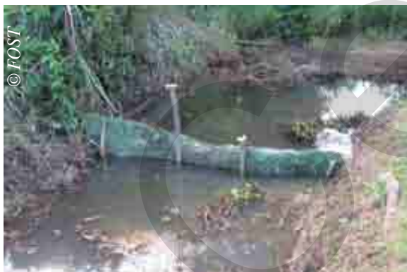
Filter barriers made of mesh and scythed vegetation
