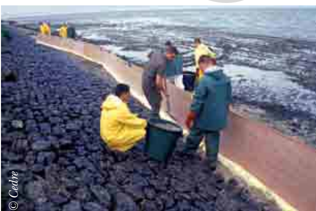
Barrier made of plywood panels to contain effluent
