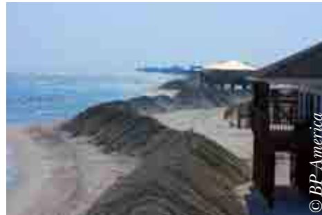
Constructing a protective dyke using loose sand, Deepwater Horizon, Louisiana 2010
