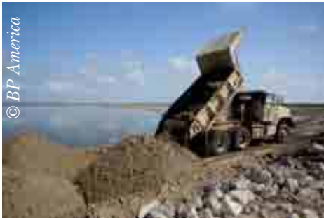
Constructing a protective dyke using loose sand, Deepwater Horizon, Louisiana 2010
