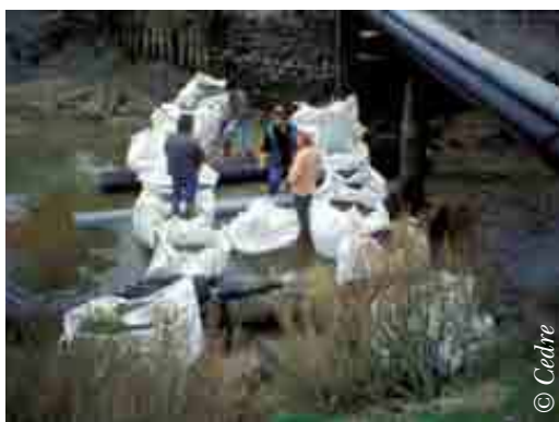
Protecting a stream using big bags and angled pipes
