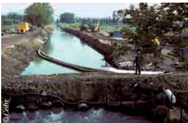
Earthen dam with pipes to let water through
