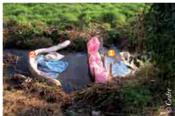
Reinforced measures: (1) filter barrier (double series of stakes with plastic mesh filled with sorbents) and sorbent boom and pads upstream (2) sorbent boom and pads
