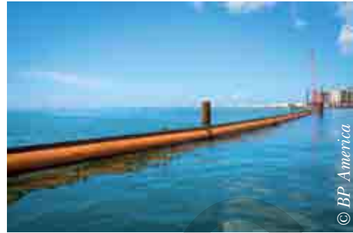
Using a floating industrial pipeline as a containment means, Deepwater Horizon, Louisiana 2010
