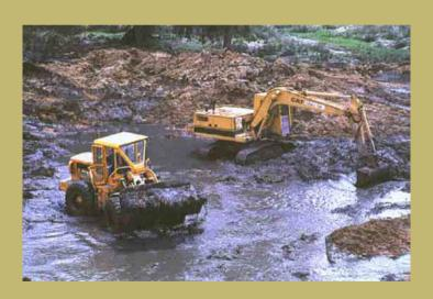
•In the cleaning works the resources employed were numerous, being simultaneously almost 500 lorries and more than 150 machines among diggers and loading machines, to remove 7 million of m<sup>3</sup> of sludge and countermined water.
