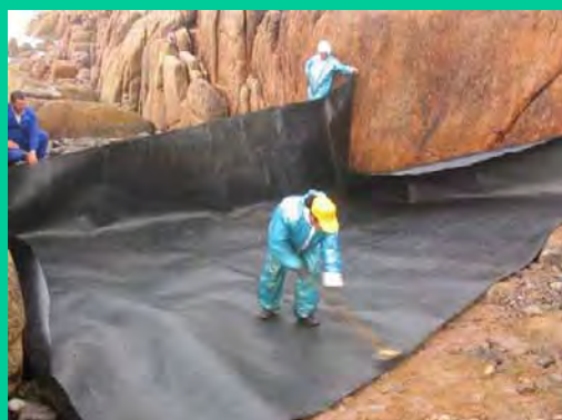
3.- Waterproofing of the bottom of the dam with a plastic liner
