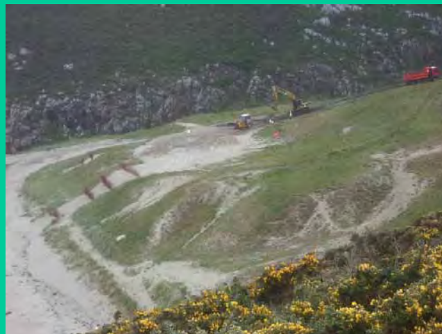
2.-Restoration of sand dunes and elimination of the provisional access road
