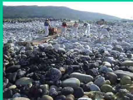
2.- Transfer of boulders using a vehicle
