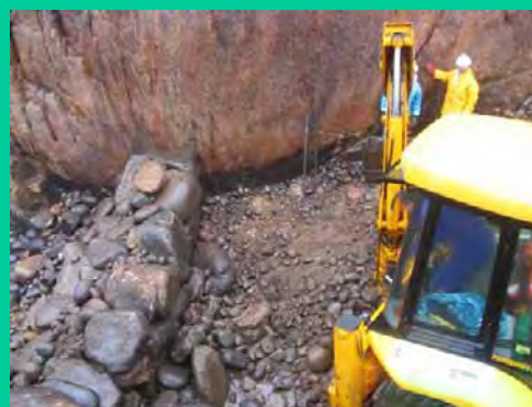
2.- Building of a small dam using heavy machinery
