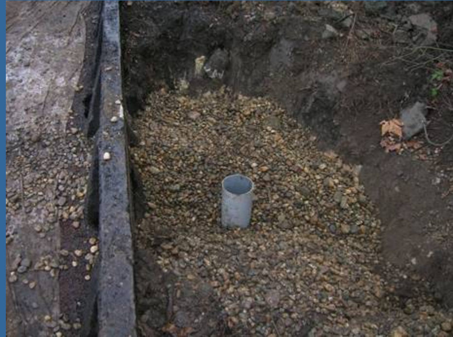
Creation of a vertical drain to conduct a spot test for pollutant soaked into the banks (began 20/01/2007)
