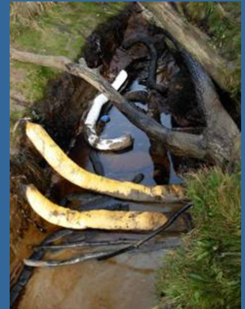
Sorbent boom deployment in front of pollutant run-off (began 14/01/2007)
