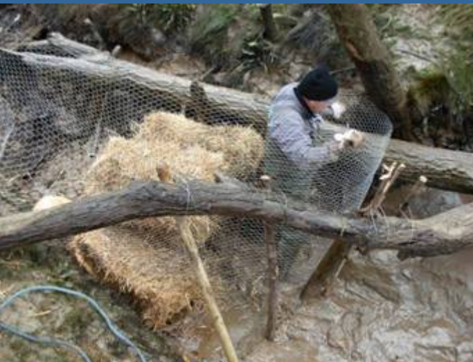
Implementation of makeshift booms (straw + wire + geotextile) to reinforce the system (began 18/01/2007)
