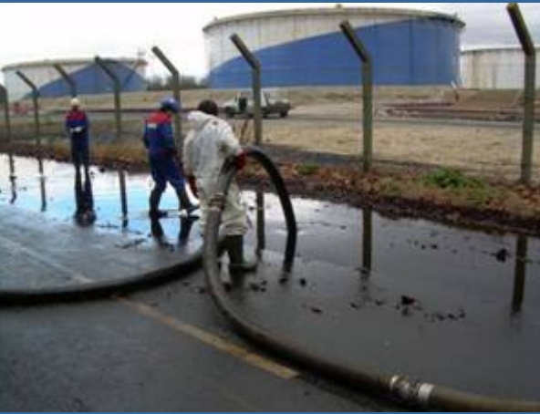
Pumping off accumulations of pollutant by the banks (began 12/01/2007)
