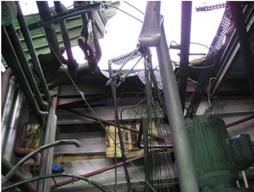
MIRECOURT (December 2006) Facility after the vertical ejection of the reactor (source: INERIS)
