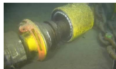
ROV view of the disconnection on the subsea gathering line (source: Husky Energy)
