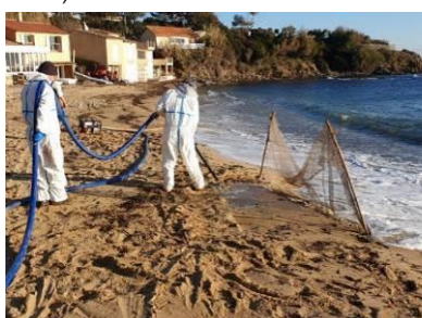
Agitation (low-pressure water jets) of sand in the surf zone to recover buried tarballs (source: LFD)
