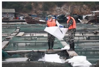
Application of sorbent mats on floating accumulations of aromatic solvent in aquaculture cages (source: www.caixinglobal.com )
