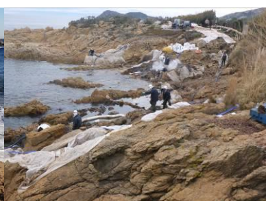
Preparation of high-pressure cleaning operations (involving effluent collection systems, protection against spattering, etc.) (source: Cedre)
