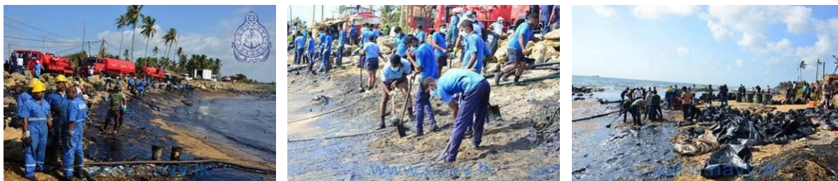
Manually recovering crude oil deposits, mixed with sediment (background: vacuum tank trucks for pumping floating oil (left); temporary storage of solid waste in bags, placed at the top of the beach (right) (source: Sri Lanka Navy)
