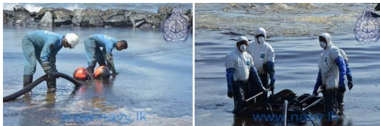
Pumping up the free oil: directly (left) or using skimmer heads (here, oleophilic discs) (right) (source: Sri Lanka Navy)
