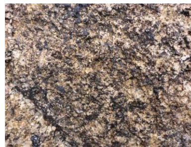
January 2019: residual traces of fuel oil after the first high-pressure cleaning operations (Casabianca / Roche Escudelier, Ramatuelle) (source: Cedre)
