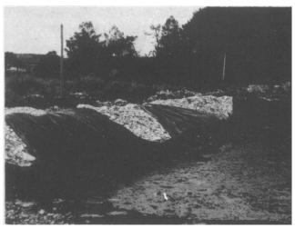
Figure 5. Temporary storage of oily residue in a lined dug pit near Roscoff
