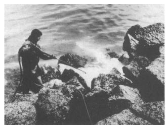
Figure 8. Cleaning of rocks using high pressure, hot water hosing technique
