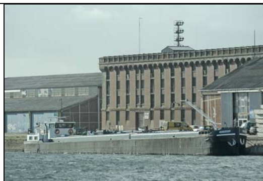
La barge Nissimus, ex-Galapagos. (source PAD)
